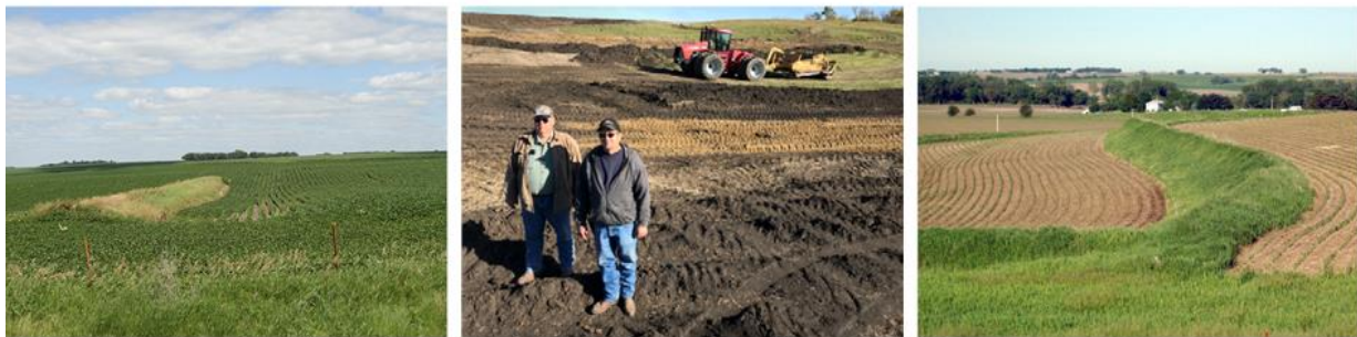
L to R: water and sediment control basin in crop field is empty in dry conditions but holds water temporarily after heavy rains; landowners pose by construction of storage basin in Pope county ag field; grass back sediment control basin slows runoff.
