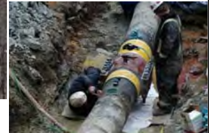
Temporary Pipeline Repair Pipeline restarted on March 23 per DOT approval
