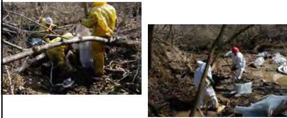
Operations removing oil-contaminated leaves and debris to increase flow through stream
