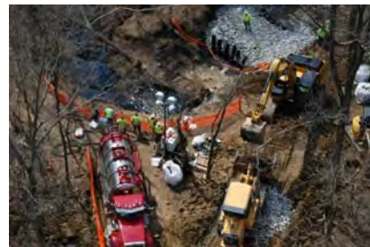
Underflow dam constructed in creek – Day 4
