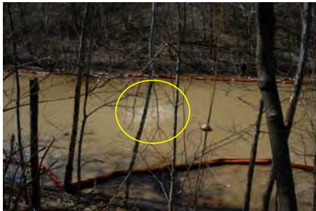
Air sparging the pond, using 3 aerators (lowers Benzene levels in water)
