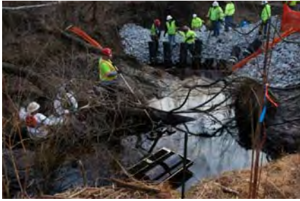
Skimming operation at underflow dam – Day 5
