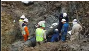
Inspecting the pipeline for damage (DOT lead)
