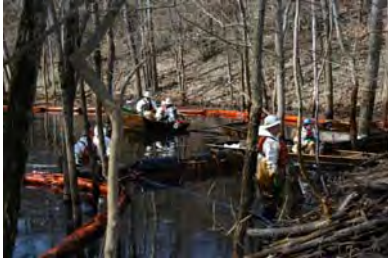
Operations collecting oil-contaminated debris and skimming oil from surface of pond
