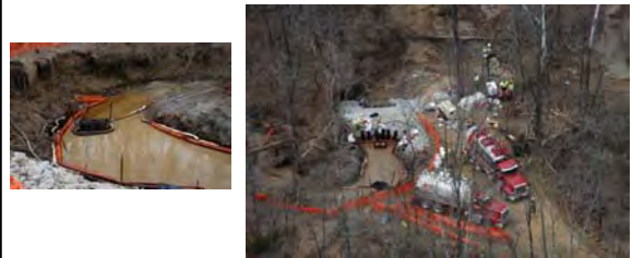
Skimming operation at underflow dam – Day 8
