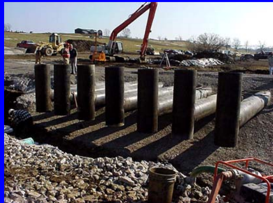
'T' Inlet allows for easy cleanout of debris
