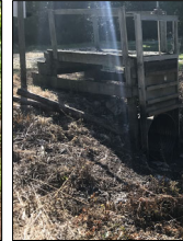
Water Control Structures
