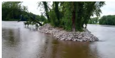
Stage 1-Huron Chute Island Erosion Protection
