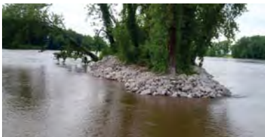
Stage 1-Huron Chute Island Erosion Protection
