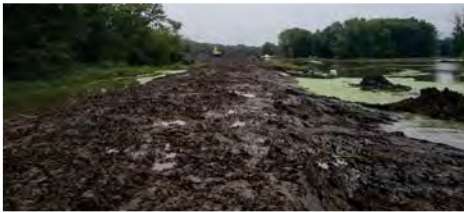
Stage 3-Kehough Slough-Upper Channel Placement and Site Shaping
